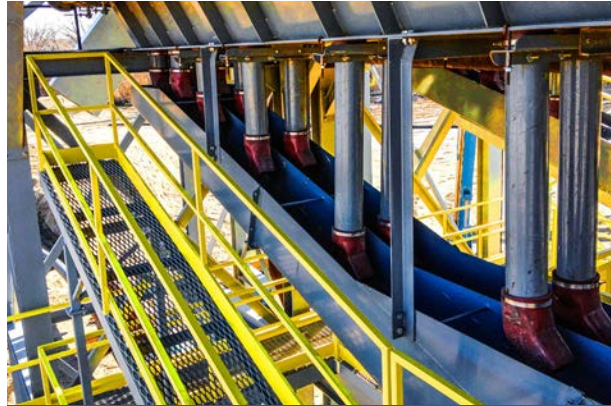
WALKWAY TO ACCESS BLENDING FLUME
