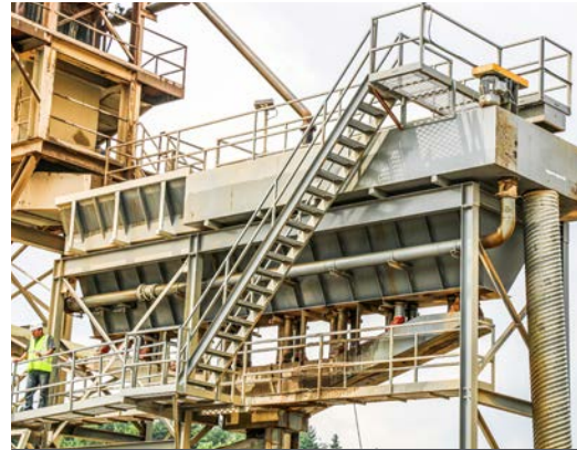
CLASSIFYING TANK WITH STAIRWAY
