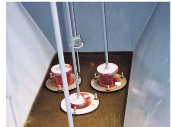
URETHANE DISCHARGE VALVES
