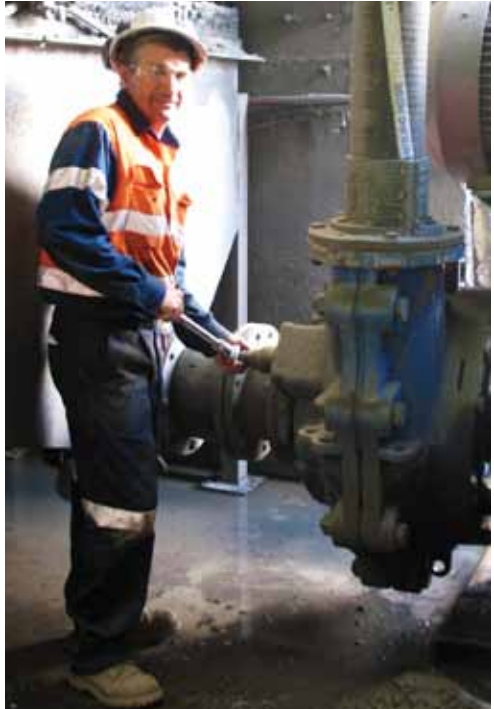
Paul Sharp from Sibelco Australia's Tallawang site in NSW, Australia, adjusts the revolutionary new Warman® WBH® pump without stopping production.
