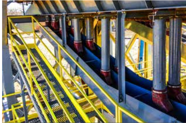
WALKWAY TO ACCESS BLENDING FLUME
