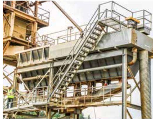
CLASSIFYING TANK WITH STAIRWAY
