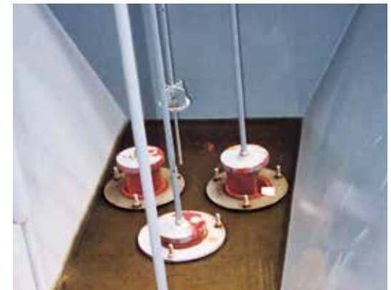
URETHANE DISCHARGE VALVES
