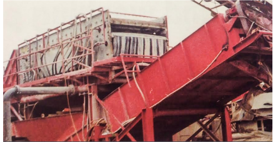
SEMI-PORTABLE WASH PLANT
