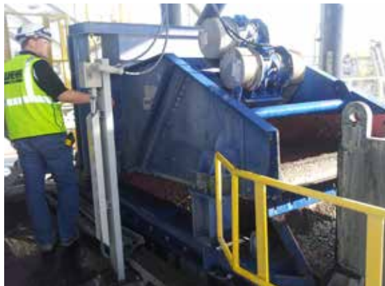
Weir Minerals expertise available on-site
